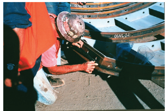
Tunnel Segment Seal
