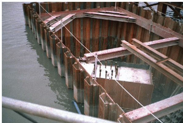
Sheet Pile Interlock
