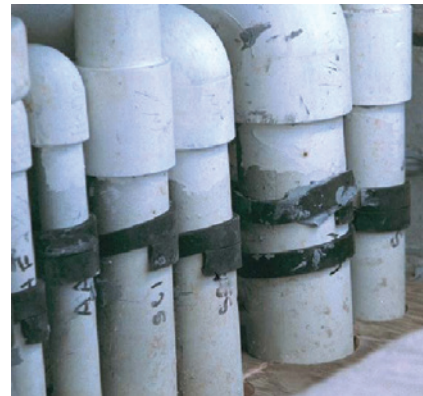
Piping Penetration
